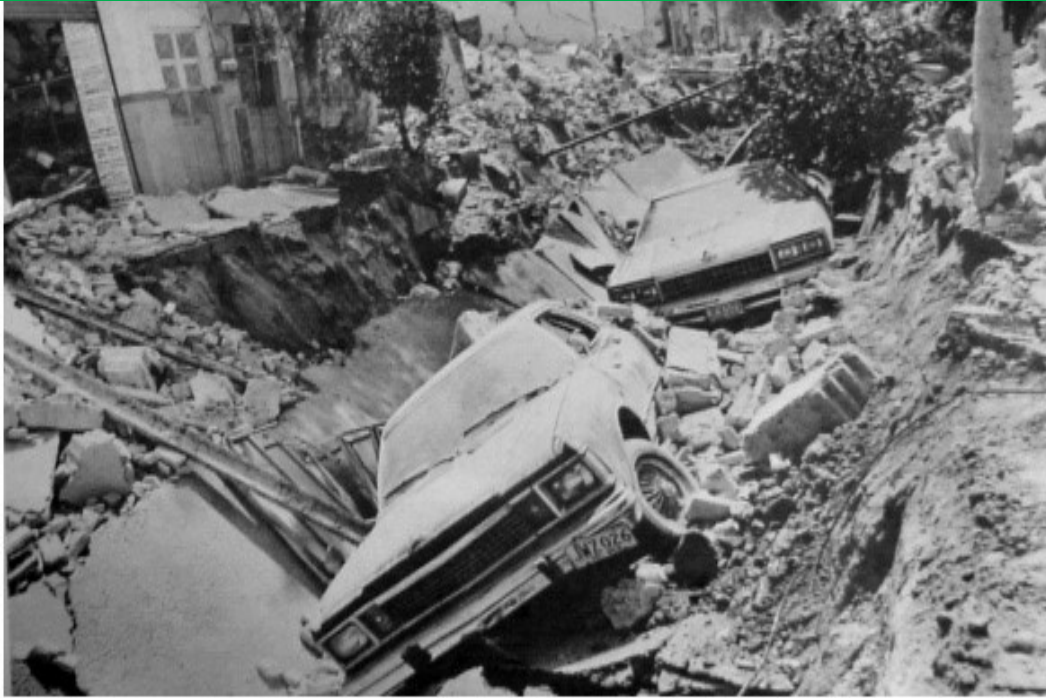
Guadalajara Sewer Explosions@1992@Mexico
