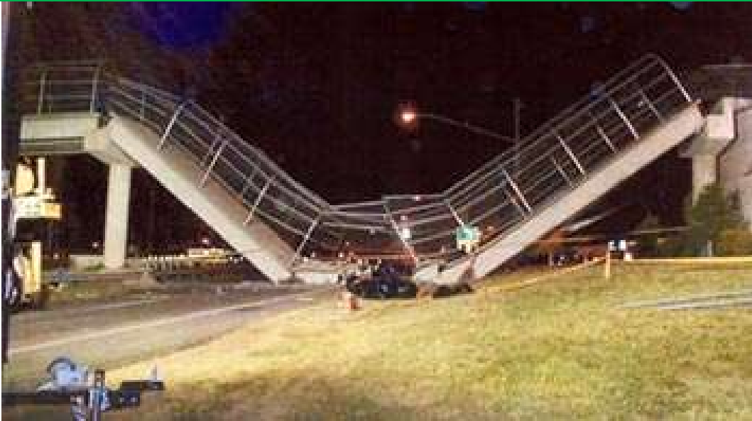
Lowe's Motor Speedway Bridge Collapse@2000@USA
