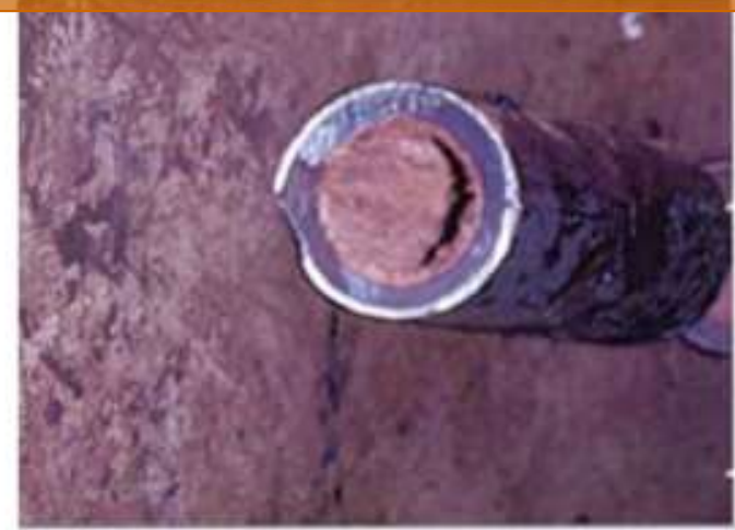
Case 1 Heavy corrosion and scaling in Monel-400 bromine preheater. (Courtesy: Elayaperumal, in "Corrosion Failures in Process Industries in India: Statistical Analysis and Case Studies" in Special Supplement 2009, Corrosion Reviews Special Issue: India, England: Freund Publications, 2009, p 51, case study 1.)
